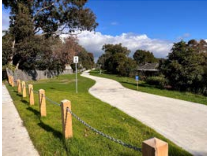
Post and chain fencing treatment controlling vehicle access
