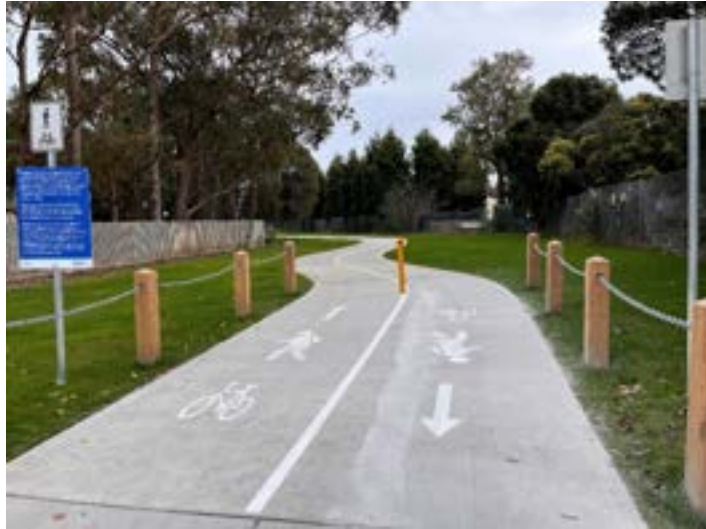
Entry treatment to shared user path (MWC M22 project)
