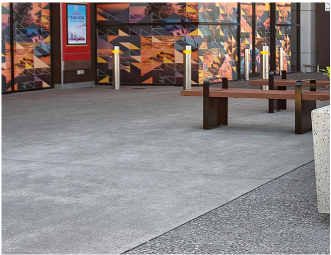
Proposed exposed aggregate and standard concrete footpath.
