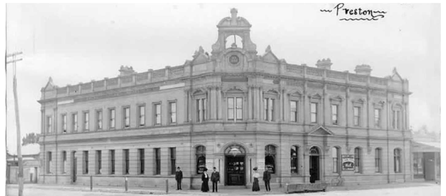
Council Club Hotel c. 1890s (formerly located on the corner Cramer and High). Image courtesy of Darebin Libraries.
