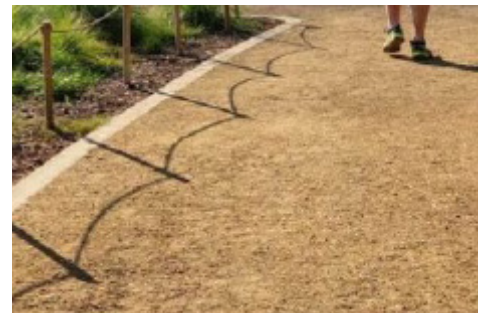
COMPACTED TOPPINGS PATHWAY
